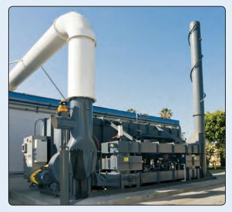
Our California facility takes pride in limiting volatile organic compound (VOC) emissions into the environment. Two regenerative thermo oxidizers are utilized to eliminate 99% of the VOC from our ventilation system before emitting air to the atmosphere.
