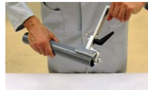
Chamfering the pipe
