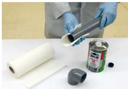
Cleaning the pipe and socket
