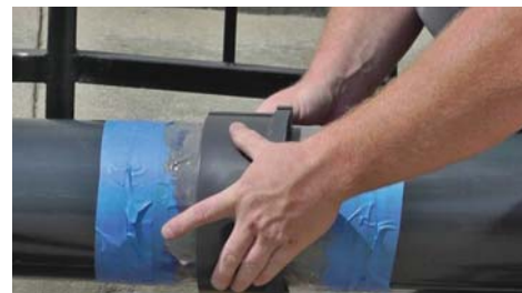
Position, Press & Hold Split Flange
